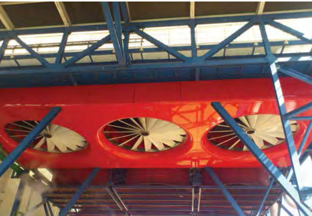
From idea to real life energy innovation, A-frame condenser with Whizz-wheel fans
